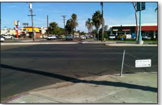
Existing Pedestrian Restricted Intersection
